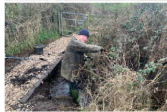
17/1/25 Haddenham bridge at SP755109 - Cleared blocked pipe
