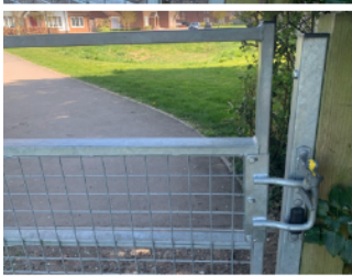
10/4/25 Pitstone at SP938162 fitted Centrewire "D" latch repair kit.
