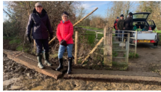
Sleepers in position and in use.
