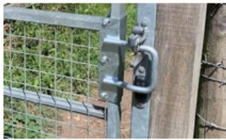
8/7/25 Waddesdon D Loop repair kit fitted at SP775134.
