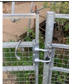
24/9/25 Haddenham D Loop repair kit fitted at SP719071.
