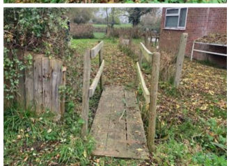
9/11/24 Westcott CAMS a02981. Cleared brambles off footbridge WES/4680 at SP720170.
