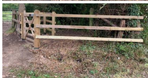
14/8/24 Return visit to Gate 350 to clear the arisings that we left behind on 31/7/24.
