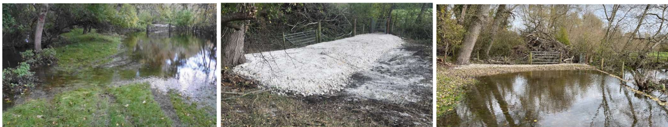
L-R: Historical photo of flooding; sub-base of chalk laid down Oct 2022; flooding Nov 2022.
