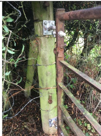
14/9/21 Rehung field gate with two new adjustable gate eyes and two new adjustable gate hooks on plates fitted to existing and retained hanging post. (254)
