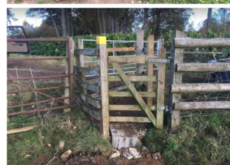
2/11/21 Cheersley CHR/10/1 at SP711109. Rebuilt timber kissing gate coral and built step.
