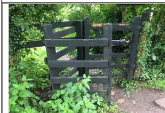
9/11/21 Cheersley CHR/10/1 at SP713108. Rebuilt timber kissing gate coral, installed gate post and fitted re- placement gate. Note Anthony Adams, far right, Cheersley foot- paths champion at- tended all three repair jobs and helped where he could.
