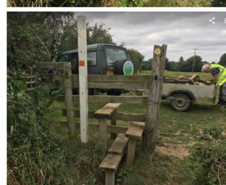
20/9/21 Dinton with Ford & Upton DFU/12/1 at SP765103. Added a third low level step and hand post to stile.
