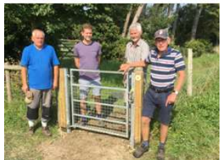
Janet's gate proved to be really difficult due to both stile posts being cemented in to full depth necessitating excessive use of the jack hammer.
