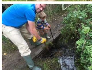
11/10/20 Haddenham HAD/5/1 at SP755100 Before & after clearing the gully blockage.
