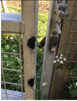
Typical photo of a failed Centrewire gate where the 18 mm solid steel hasp has broken at its two welds to the 1 mm thick channel section.
