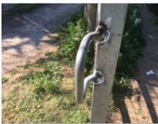
25/4/20 Haddenham HAD/19/1 at SP100737. Weld repair on "D" latch.
