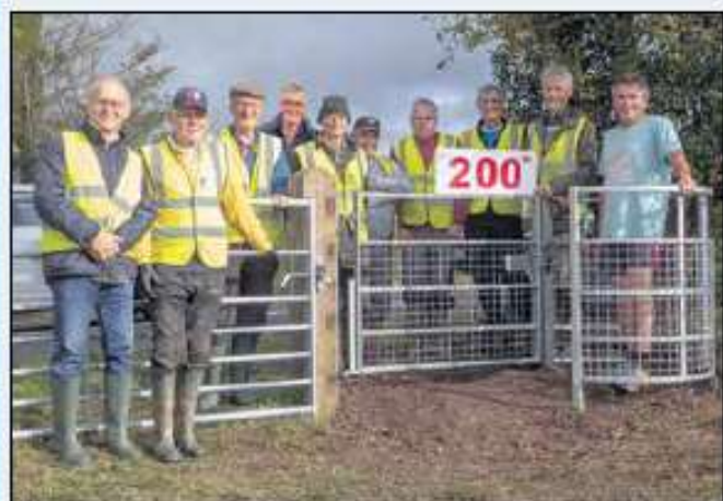
One less stile to cross: The installation team with their 200th gate which was donated by Stone, Haddenham & Dinton's Simply Walk group.
