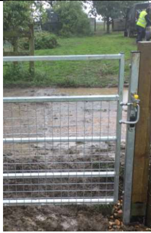
25/6/19 Oving OVI/6/2 CAMS 88806 at SP793230 NOT completed. Gap on other side of track instead.
