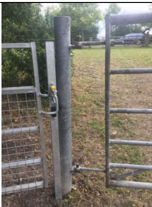
9/7/19 Ford. At Gate 172 rehung the field gate with two extra long eye bolts as the steel posts had splayed excessively. FOC for Chris Woods.
