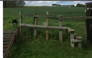
175 mm diameter strainer post to left of our usual 1.8 m x 100 x 100 gate post. Livestock warning notice rescued by Andrew from the stream and attached to leaning sleeper.
