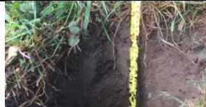
910 mm depth for strainer posts.
