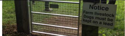
175 mm diameter strainer post to left of our usual 1.8 m x 100 x 100 gate post. Livestock warning notice rescued by Andrew from the stream and attached to leaning sleeper.
