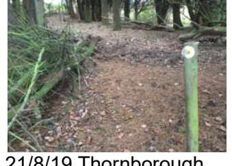
21/8/19 Thornborough THB/6/4 at SP739322. Fallen tree cleared using chain saw.
