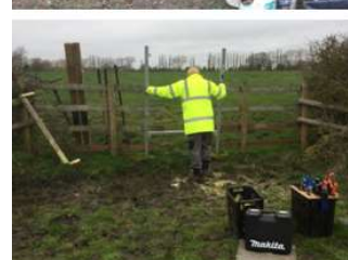
20/3/19 Westcott "Work in progress" on both sites – three S2Gs.
