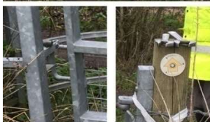
12/12/18 Shabbington SHB/9/5 at SP663073. Adjusted latch so gate would self-close properly.
