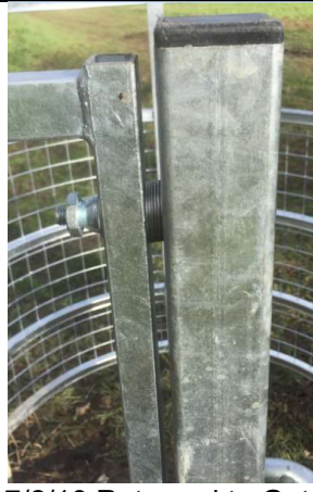
7/2/19 Returned to Gate 149 to insert a number of washers to stop "H" from splaying.
