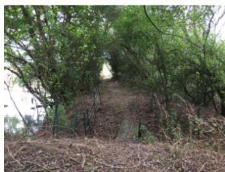
11/9/18 Oving OVI/14/3 at SP788229. Vegetation clearance.
