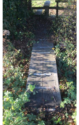
21/11/18 Westcott WES/28/2 at SP720165. Added 3 anti-slip strips each with 3 screws.
