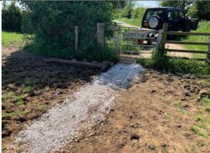
20/5/24 Haddenham HAD/5/1 at SP751098 Surface Improvements CAMS a01767. Paving slabs removed.
