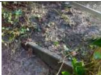
6/12/23 Fitted a pro- tective metal strip to step installed by John on 28/11/23 at Gate 338.
