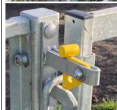
22/1/24 Refitted yellow latch that had mysteri- ously fallen on the ground. Fitted a tam- perproof security nut.
