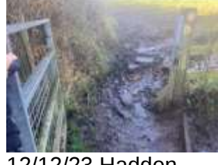
12/12/23 Hadden- ham HAD/5/1 at SP755100. This per- ennially muddy and slippery slope has been referred to Bucks RoW team.
